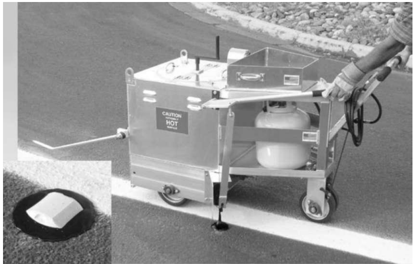
MANUALLY OPERATED AGITATOR AND MATERIAL TEMPERATURE INDICATOR
